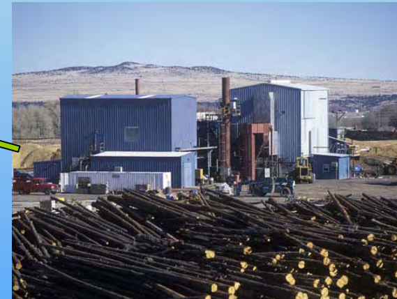
3 MW BIOMASS PLANT EAGAR, ARIZONA
