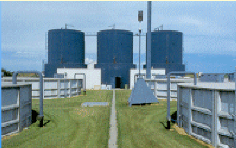
Lemvig centralised biogas plant, Denmark, producing about 4 million m 3 /year of gas Agores Website
