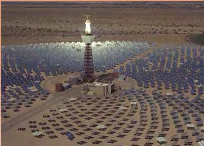
10 MW Solar II Experimental Power Plant, California
