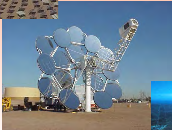
25 kW Dish/Stirling Engine System, Arizona
