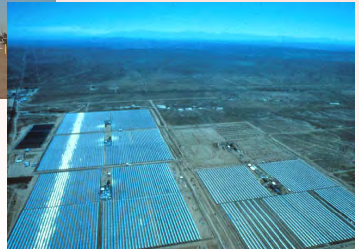
350 MW Parabolic Trough Power Plant, California
