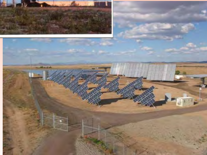
Prescott Airport, Single Axis, Tilted Tracker Single Axis and High Concentration Photovoltaic
